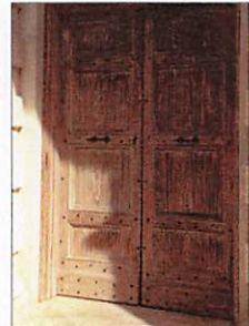
STAINED WOOD DOORS & GATES WHITWASHED CYPRESS
